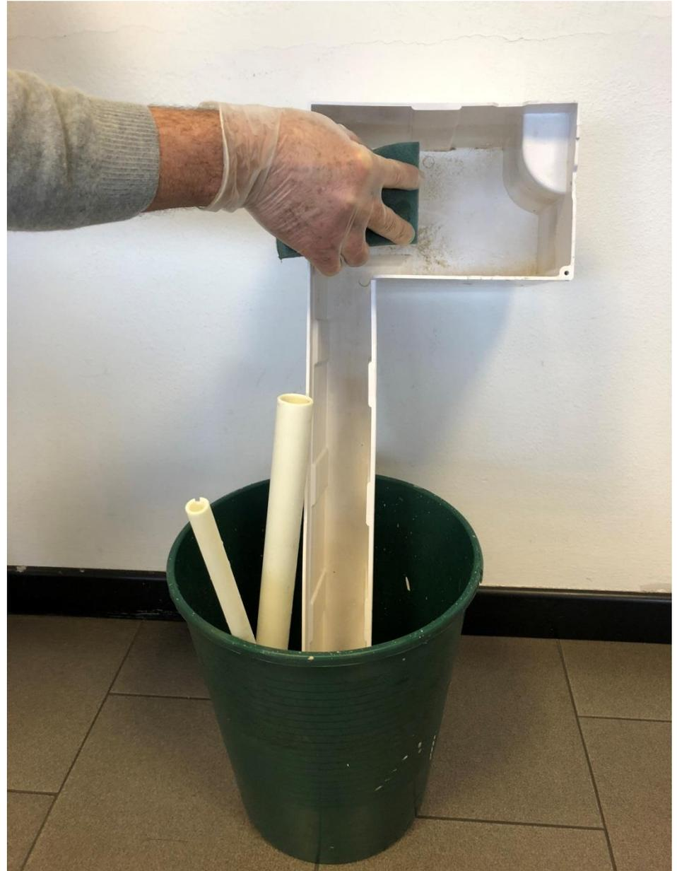
All above step (cleaning) shall also be made by antibacterial solution (finally rinsed by fresh water) then, carefully reinstall all cleaned removed parts
