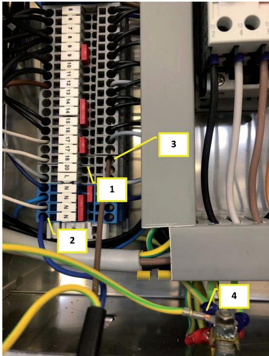
1. Remove jumper from contact 17 and 18 of the machine terminal board.
