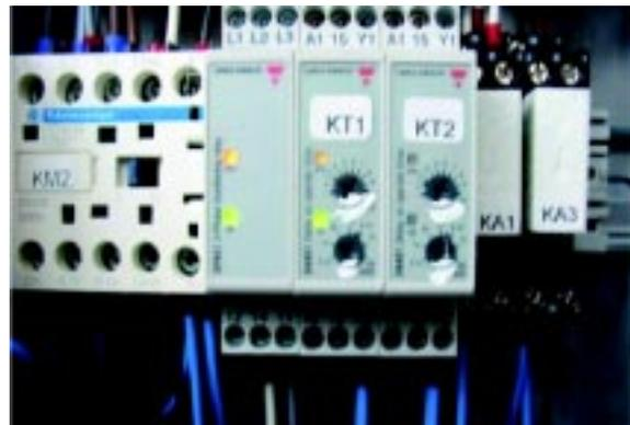
**NOTE.** In case on any temporally Ice maker trip OFF (not alarm) due to NO/LOW water pressure, bin full, ice spout switch activation unit stops by only keeping drive motor operating for 18' in order to clear evaporator by ice. KT2 delay relay LEDs steady ON (orange and green) during this delay.
